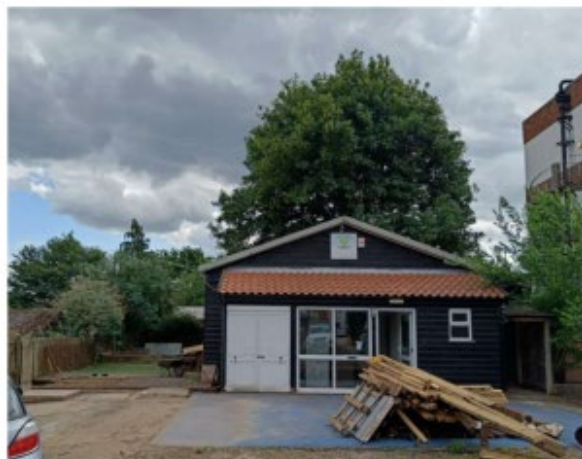
Figure 3: North facing elevation of the building.
