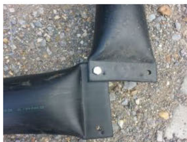
1. Bolt the corners together using stainless steel fixings
