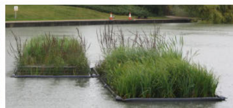
6. Your island is now ready to push in to place on to the water and then secure to the anchor weight
