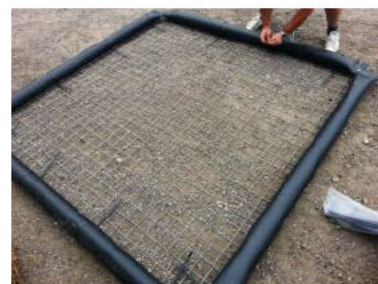
2. Place mesh base underneath booms and secure with heavy duty cable ties as shown
